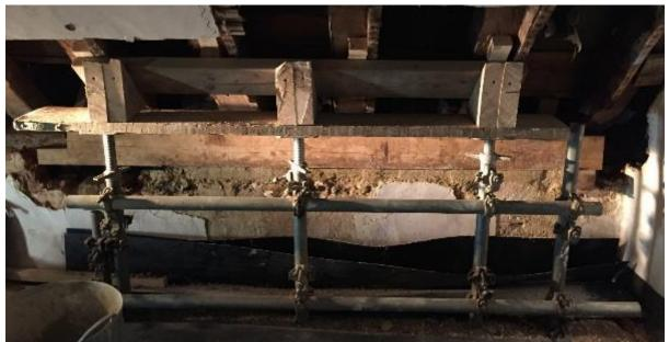
The southern end, visible externally – it is a tight fit. Here, the shorter Northern section has been added and jointed to the remainder of the existing plate.
