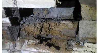
importantly, moisture content in the wood at 12-15%, was too low for a current infestation. We have the tiled roof replacement of 1968-9 to thank for that.
