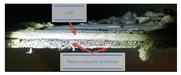
On removing the board, we discovered the ceiling condition might be worse than feared.
