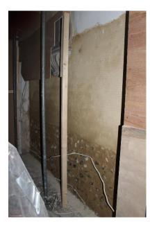
In this photo, from the North wall, the untouched white wall can be seen at the top, the middle section is freshly re-plastered and the bottom, normally hidden behind the choir pew, has been scraped out and repointed.
